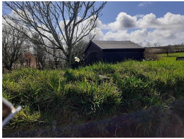
Existing Shed on Site
